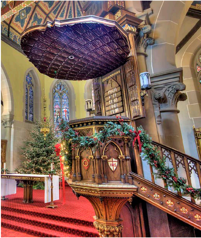
Figure 4. Notice that the sound board has carvings of plants on the underside of it oriented front to back. This is the proper way to apply diffusion to assist with speech.
