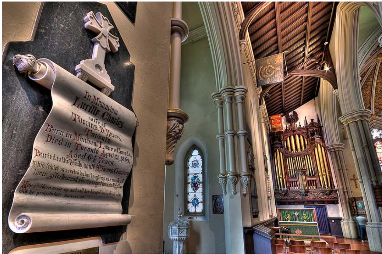
Figure 6 There are eight features in this photo that helps to tame the sound in this church. (1) Marble memorial, (2) the beveled window frames, (3) the pillars, (4) the rounded shapes on the pillars, (5) the pipe organ, (6) the coffered wood ceiling (7) the crown molding to cover the connection from the wall to the wooden ceiling (8) the open wood trusses. It is the sum of all of the parts that makes this room work. St James Anglican Church, Toronto, Ontario, Canada. Photo by Joseph De Buglio
